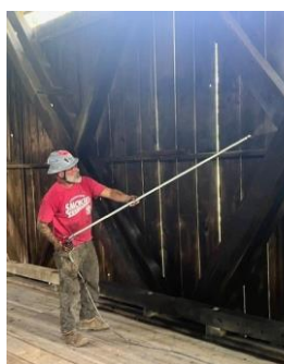
Brown Bridge OH/35-08-04 Application of Fire Retardant
